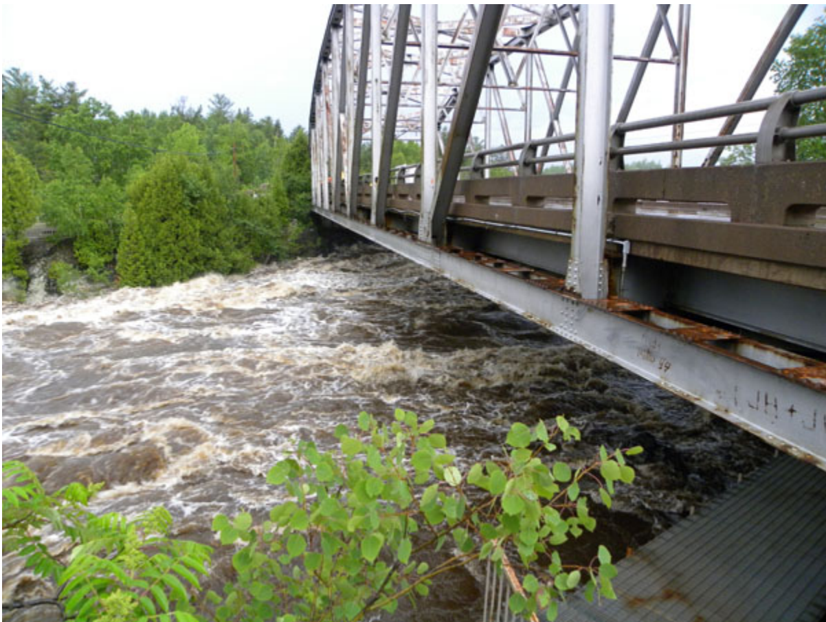
The St. Louis River flows under the Hwy 210 Thomson Bridge. Photo by Tom Lund
