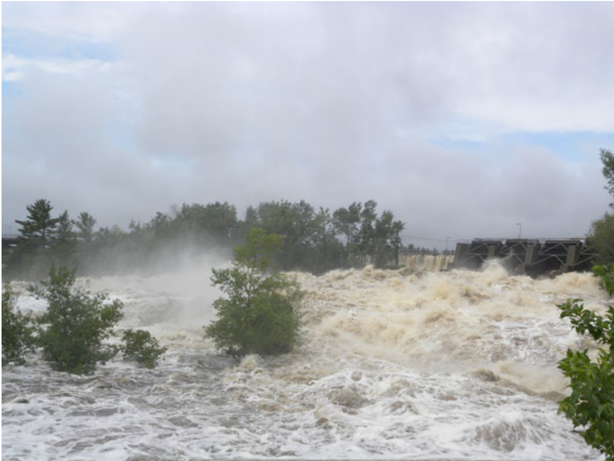
The St. Louis River rages near the Hwy 210 Thomson Bridge southwest of Duluth. The Thomson Dam can be seen in the background. Photo by Tom Lund
